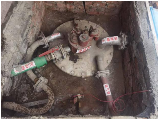
油罐区一侧静电释放桩
