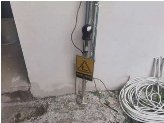
油罐区一侧静电释放桩
